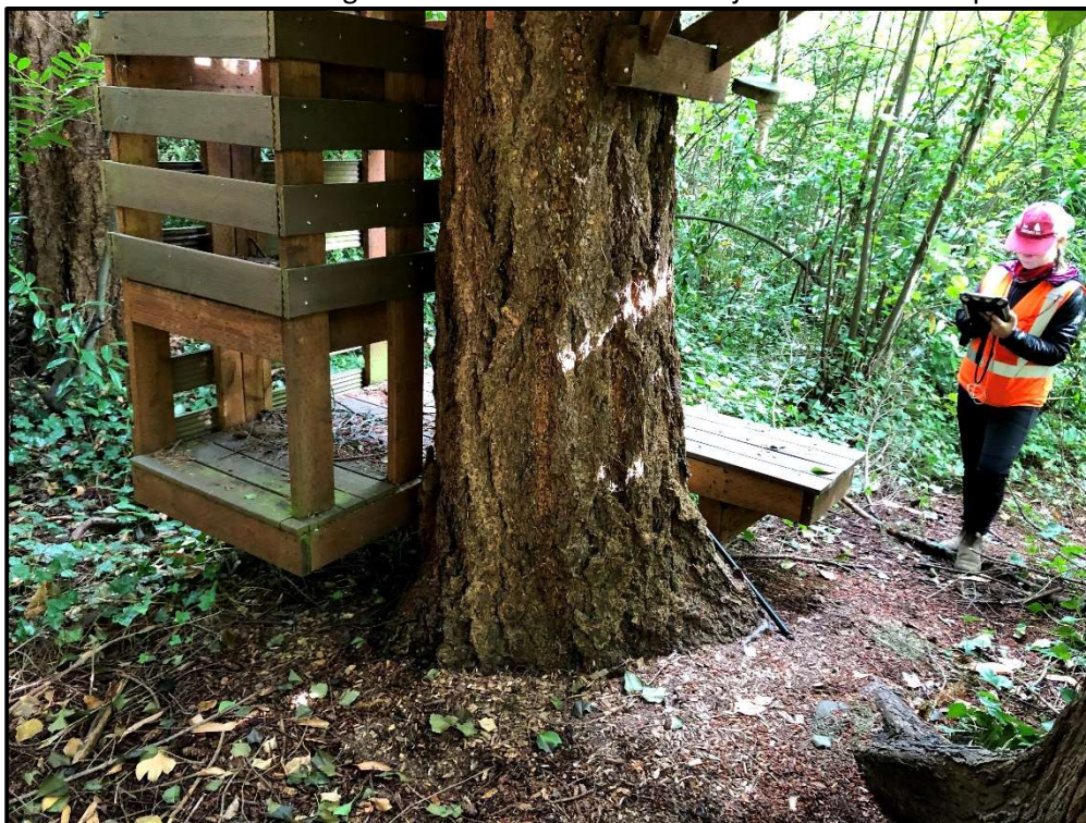
Photo 4. Tree 1810 has a platform and ladder with swing and zipline attachments; it is a primary support for the structures.
