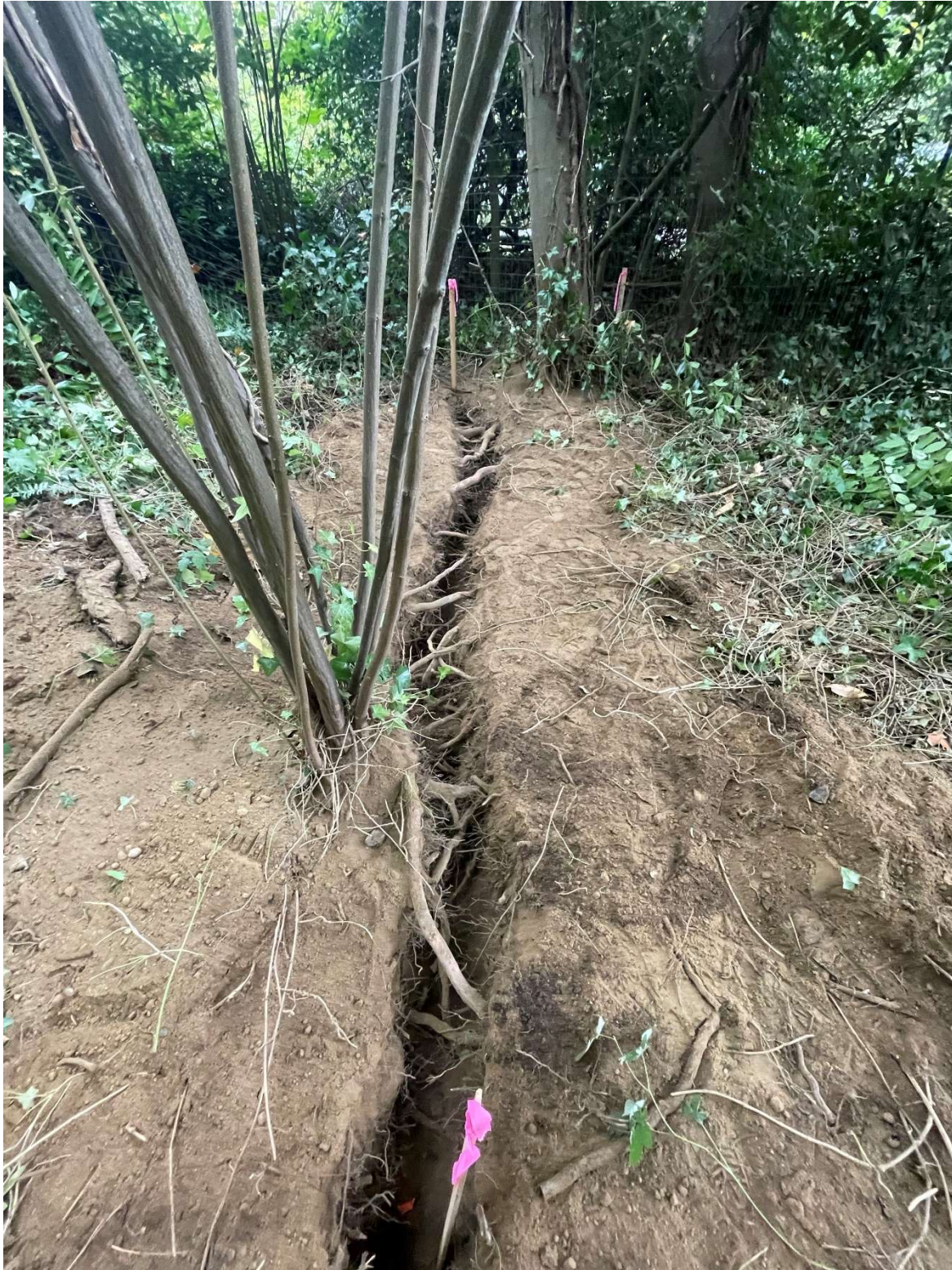
Photo 8. A closer view of roots encountered during air excavation at the edge of the proposed walkway. All visible roots are associated with the non-regulated beaked hazelnut or red alter tree 1814, which is proposed for removal.
